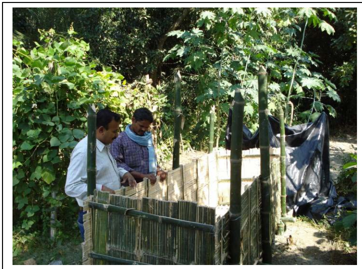
A bamboo vermicomposting unit under construction.
